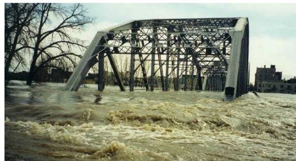
Photo: U.S. Army Corps of Engineers
