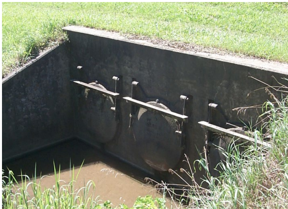
Photo: U.S. Army Corps of Engineers
