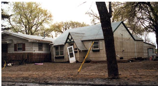
Photo: U.S. Army Corps of Engineers
