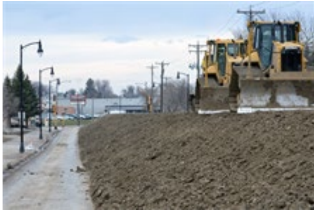
Photo: U.S. Army Corps of Engineers
