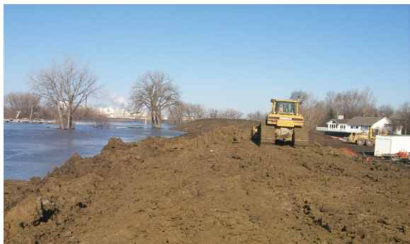
Photo: U.S. Army Corps of Engineers
