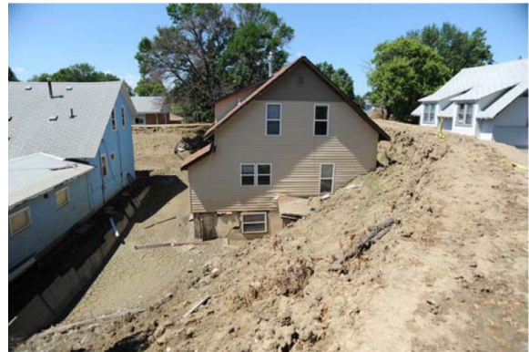
Photo: U.S. Army Corps of Engineers
